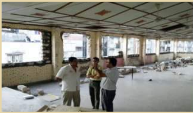
Photo 7: Renovation Work in Progress
