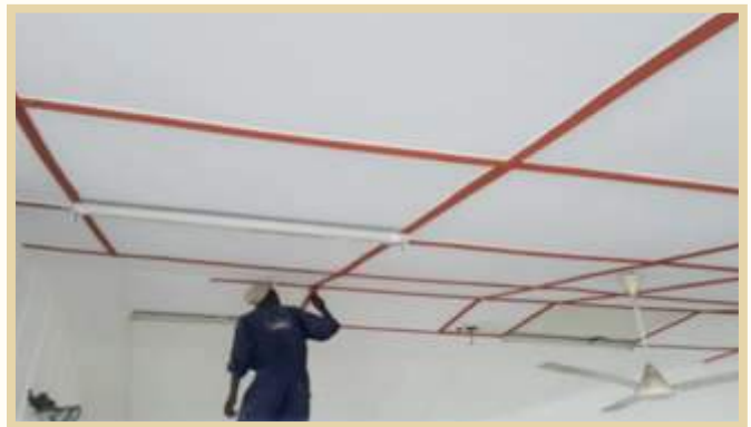
Photo 5: Paint work in progress
