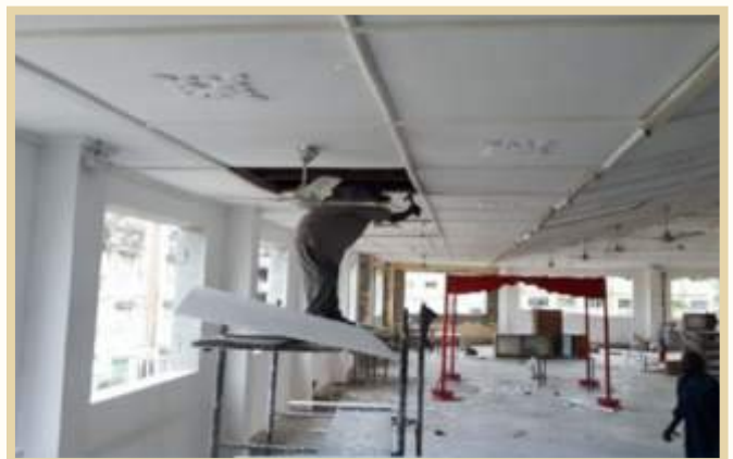
Photo 4: Ceiling board repair work in progress
