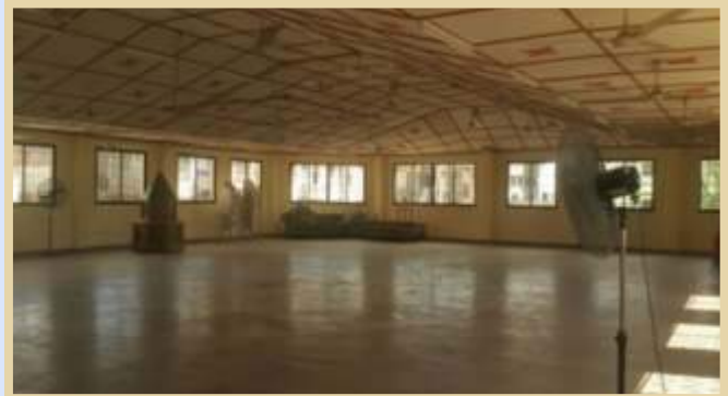
Photo 10: Rear View after Renovations
