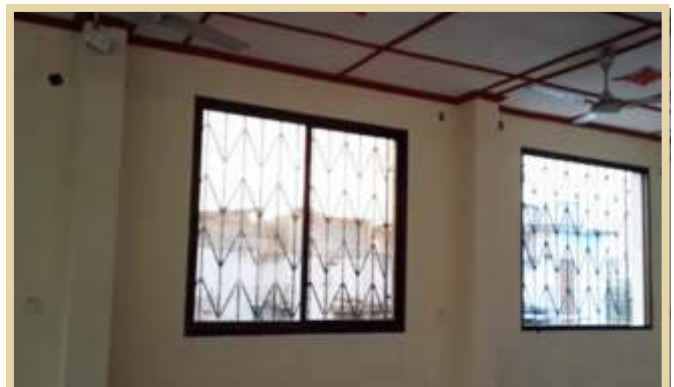
Photo 6: Sample Aluminium window fitted
